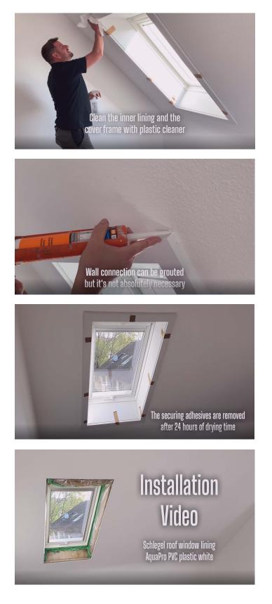
1. Clean the inner lining and the cover frame with plastic cleaner (for real wood inner lining with a damp cloth).
