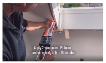
4. Foam all four foam points with fast-curing 2K PU foam.
