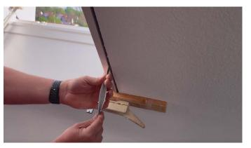
3. Insert strips of paper or newspaper at all four foam points. This distributes the foam optimally and prevents it from dripping onto the floor.
