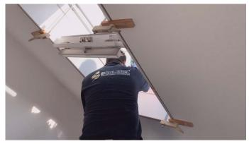
1. Insert lining box into the groove of the roof window frame on the insulated roof window.
