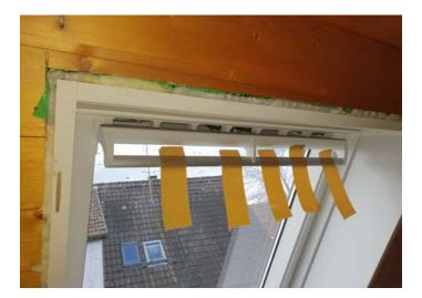
The lining is firmly installed in the roof with 2K foam (yellow foam). For insulation, the 1K PU foam (grey foam) is inserted in the front area.
