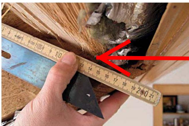
Leave some distance to the rafter so that the installation can be carried out without problems.
