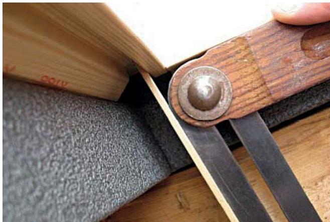
Place the angle measuring tool on the lower corner. Place the metre rule on the angle to simulate the material thickness.
