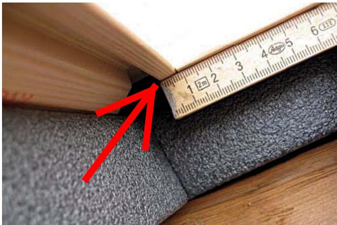
Place the metre rule on the inner edge of the roof window groove.
