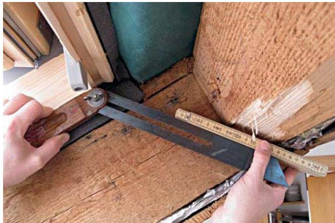
Place the angle measuring tool at the upper corner. Place the metre rule on the angle to simulate the material thickness. Raise the angle so that the cover frame covers sufficiently.
