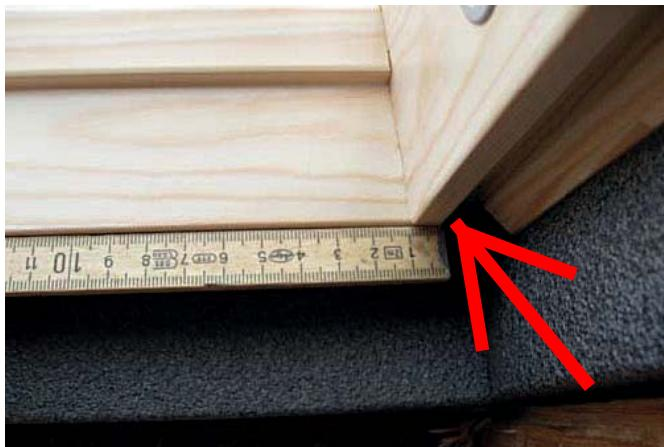
Place the metre rule on the inner edge of the roof window groove as before.
