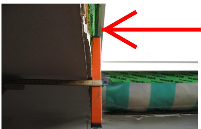
Then measure the frame width from the inner edge of the roof window groove with the metre rule.
