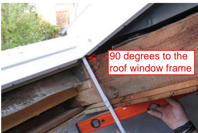
Place the metre rule at the bottom from the corner of the roof window groove at **90 degrees to the roof window frame**, then measure the dimension including the groove depth to the front edge of the ceiling.
