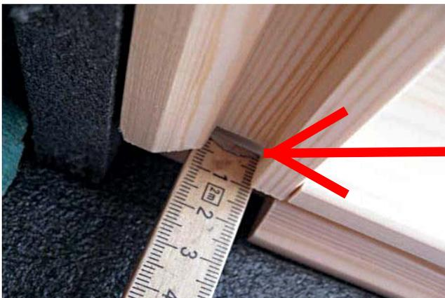
To compensate for unevenness on the ceiling, subtract approx. 4 mm in the groove from the total lining depth.
