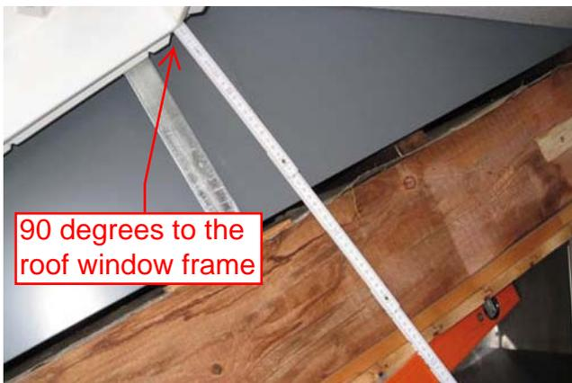
Place the metre rule at the top from the corner of the roof window groove at **90 degrees to the roof window frame**, then measure the dimension including the groove depth to the front edge of the ceiling.
