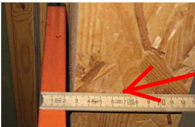
The standard widths of our cover frames are 65, 80 and 100 mm.
