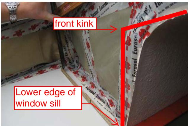
With surrounding frames, the window sill is flush with the wall. In the case of attached frames, there is a projection of at least 3 cm over the wall.
