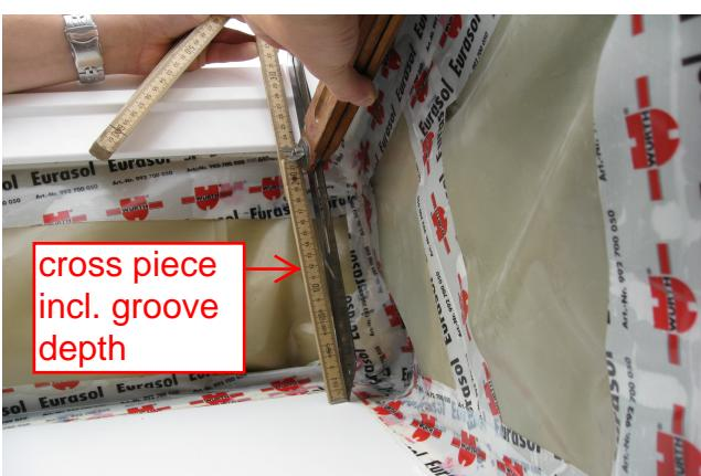
Measure the **cross piece including the groove depth** to the lower edge of the window sill. Leave a gap of at least 1 cm at the bottom so that the lining can be installed without problems.
