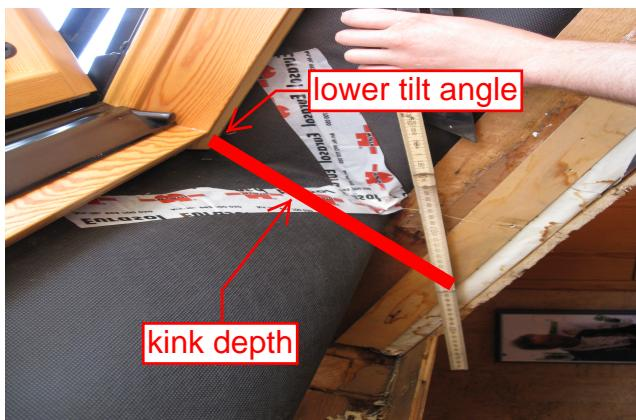
Measure the **lower tilt angle** (usually 90 degrees) and the **kink depth** with the metre rule.
