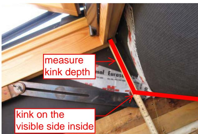
Measure the **kink depth** incl. groove depth. The measurement gives the depth of the kink on the **visible side inside!**
