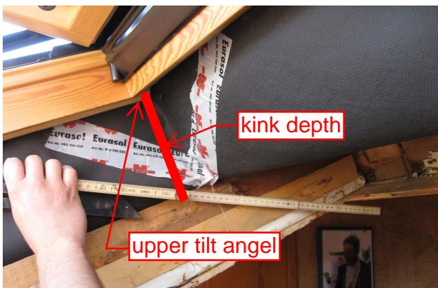
Measure the **upper tilt angle** (usually 90 degrees) and the **kink depth** with the metre rule.
