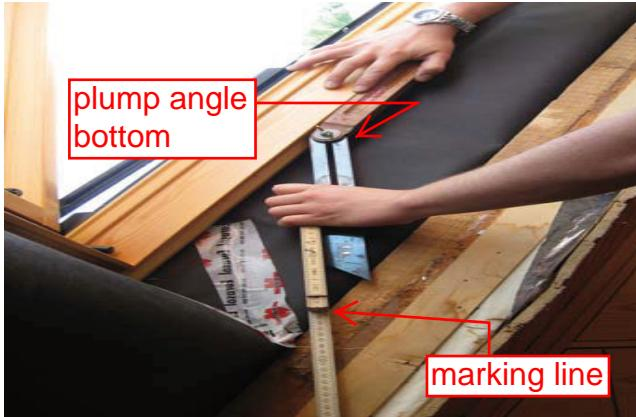
Adjust the angle measuring tool on the roof window frame so that the cover frame covers the bottom sufficiently. It is advisable to draw a **marking line** on the rafter or on the insulation foil. Then measure the **plumb angle bottom**.
