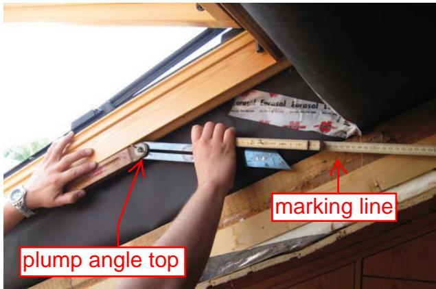
Adjust the angle measuring tool on the roof window frame so that the cover frame covers the top sufficiently. It is advisable to draw a **marking line** on the rafter or on the insulation foil. Then measure the **plumb angle** at the top.
