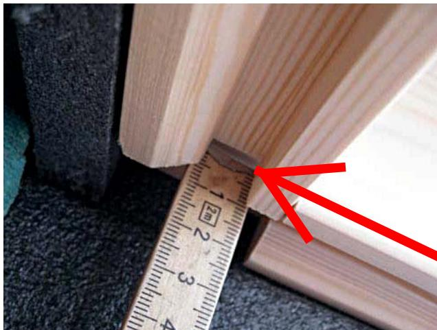
Measure the depth of the lining at all 4 corners up to the ceiling.
